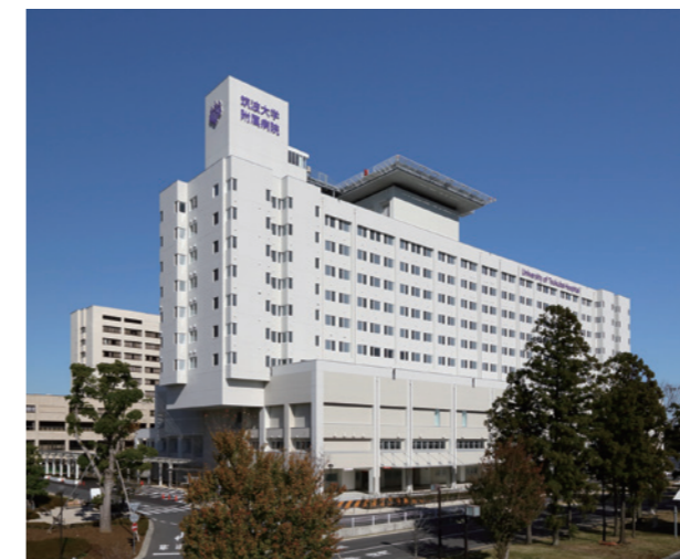
An exterior view of the University Hospital
